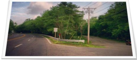
Original alignment on right in Brimfield
